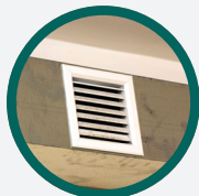
Dust from new construction and air vents
