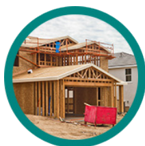
dust new construction
