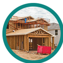
dust new construction
